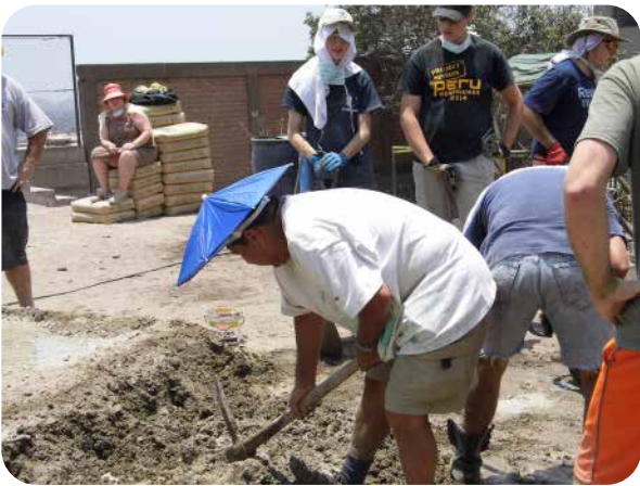
Construction of concrete stairs leading to the Oscar Romero Center
